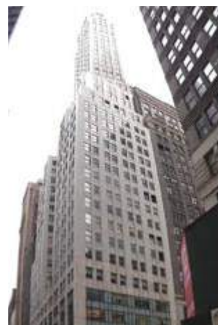
FUJITSU GENERAL SOLUTION CENTER "THE AIRSTAGE" (Stany Zjednoczone)
